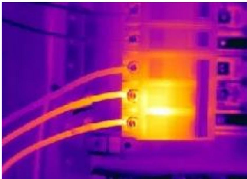
Figure 51. Image of a Compact Switch Thermal
