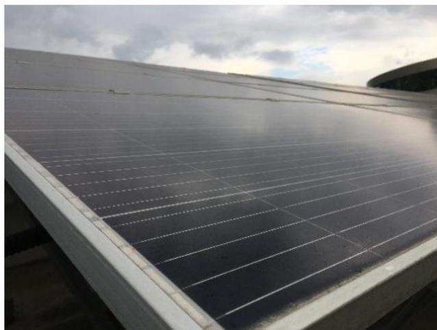
Figure 38. Polycrystalline Solar Panel
