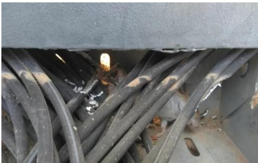
Figure 50. Insulation Errors
