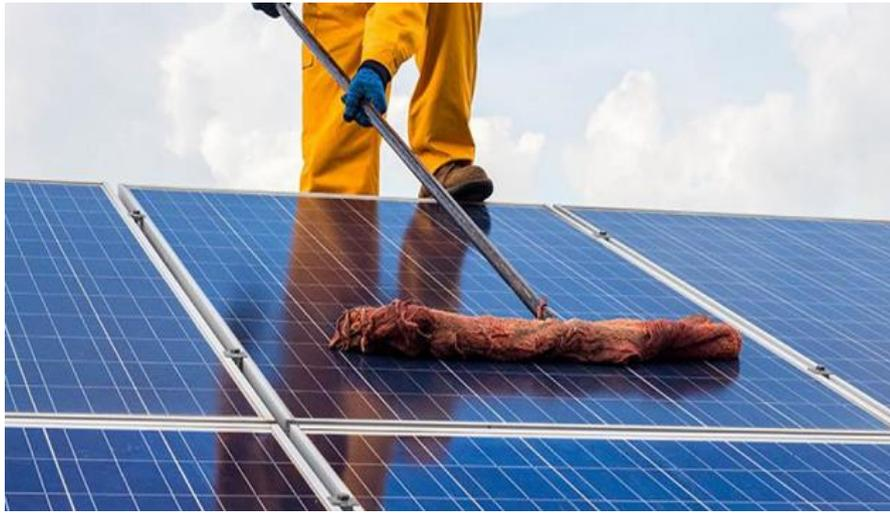
Figure 55. Manual Panel Cleaning
