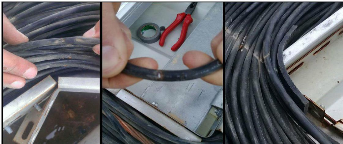
Figure 61. Cable and Cabling Damages
