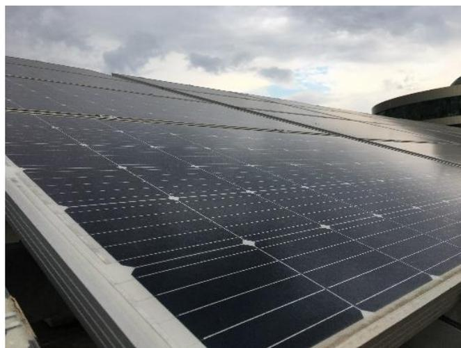
Figure 37. Monocrystalline Solar Panel
